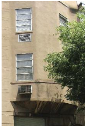
Left: Permastone and stucco cover original brick
