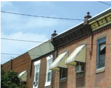
The Tale of Four Cornices: This photo shows the evolution of the ornamental cornices on a row of houses in South Philadelphia. On the right are two original painted metal cornices, one painted two colors to highlight the detail. The middle cornice was covered with vertical aluminum siding; the cornice had probably deteriorated or perhaps the homeowner was tired of painting and wanted a "facelift". At the very left, the entire cornice has been removed; only the brick remains. This original brick was laid up with texture for attaching the cornice.
