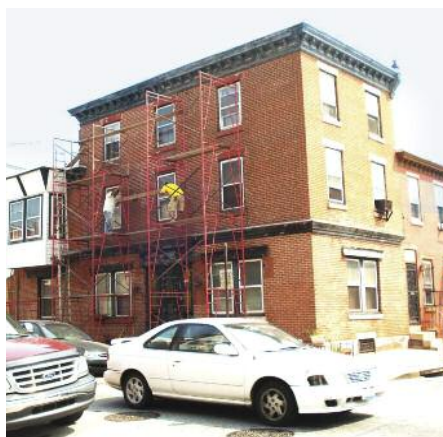
A renovation underway in Gray's Ferry
