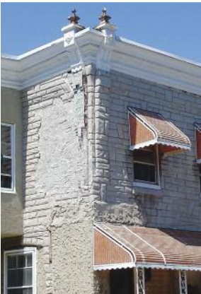
Left: Permastone and stucco cover original brick
